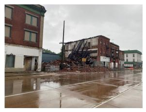
August 11, 2023, the structure located at 1006-1008 S 4th St collapsed causing damage to the adjoining structures on the 1000 Block of S 4<sup>th</sup> St. A structure engineer viewed the structures and recommended that all the buildings be demolished immediately due to danger of possible further collapse.
